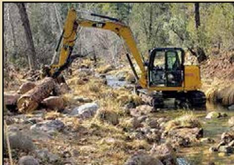
An excavator was used to lock in large boulders to create pools and embed log barbs into the eroding bank to create great habitat, while protecting the bank from erosion.
